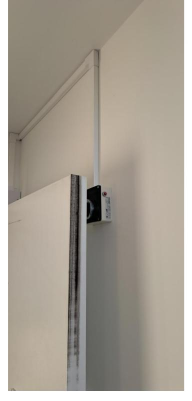
Suitable fire action notices installed. AOV system and unit inspected and deemed satisfactory. Escape route fire doors include suitable audio-magnetic hold-open devices.
