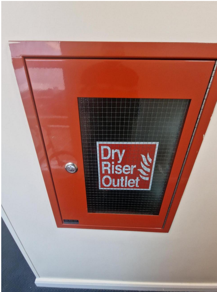
Dry riser installation.
