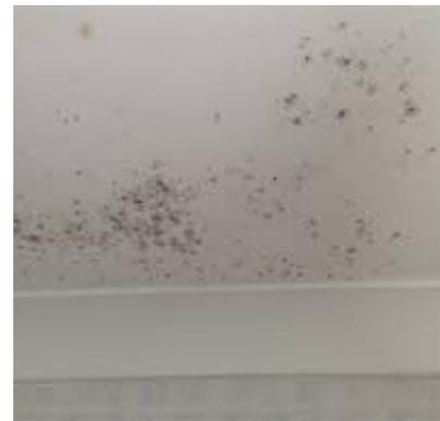
These images show examples of condensation, and mould caused by condensation
